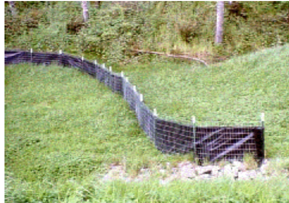
Figure 6—Silt Fencing for Sedimentation Control (courtesy of O'Brien & Company)
