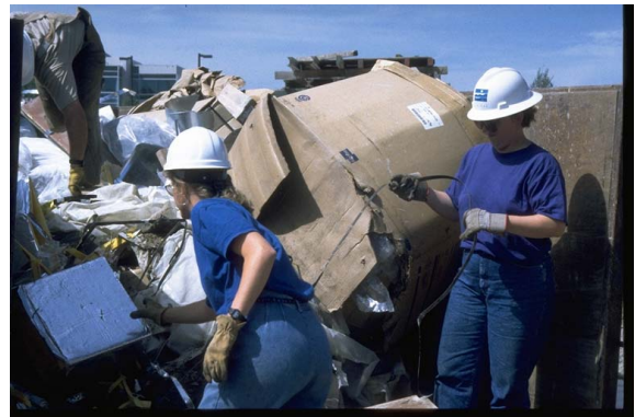
Figure 4—Conducting a Construction Site Waste Audit (courtesy O'Brien & Company)
