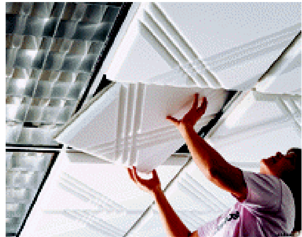
Figure 39—Acoustical Ceiling Tiles
