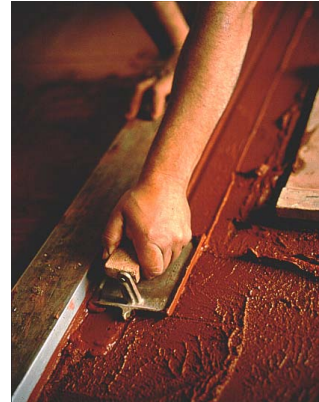
Figure 30—Installation of Finished Concrete Flooring
