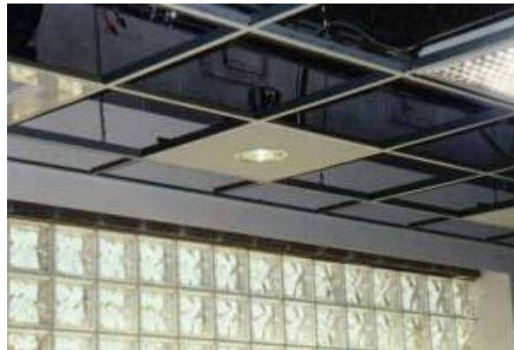
Figure 34—Acoustical Ceiling Tile/T-Bar Installation
